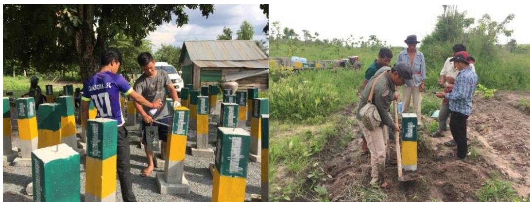
Figure 4. Production and installation of the corner posts
