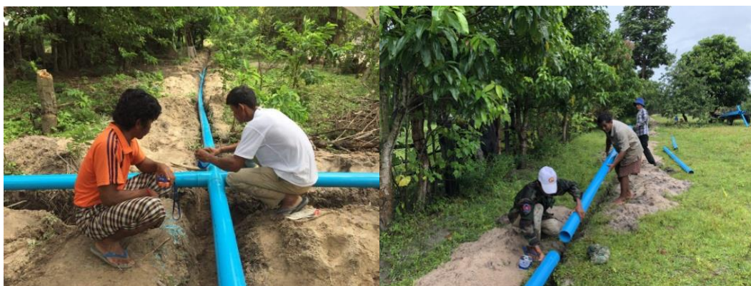
Figure 25. CF members laying out the water pipes
