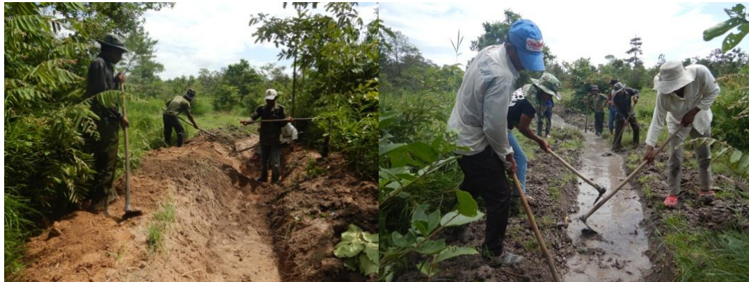
Figure 18. Drainage canal constructed in the restoration site
